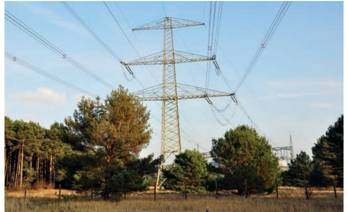
Trees in vicinity of a power line route
